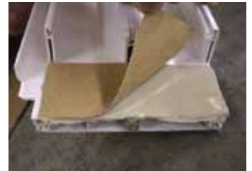
Correct placement of reinforcement.
