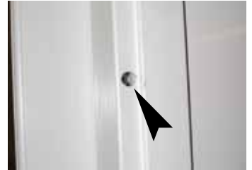
Pre-drill holes into panel through two-stepped holes in astragal.
