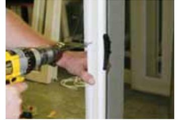
**26** Install screen lock keeper onto screen astragal.
