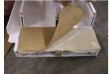
**4** Attach each jamb to the sill and head with three (3) #8 x 2-1/2" pan head screws through pre-drilled holes. Start screws in each pre-drilled screw hole by hand to assure proper screw alignment and prevent damage to the gasket. Be careful that you do not over tighten the screws, which could damage the frame.
