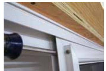
**25** Install screen astragal onto screen, using supplied screws.
