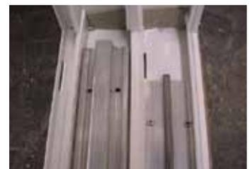
**NOTE:** Remove roller track from the sill before pre-drilling the screw holes to prevent accidentally drilling completely through the frame.
