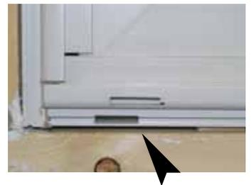
**30** Finish off the installation of the door's interior by loosely inserting insulation between the door frame and the opening. Do not over pack the insulation or the frame could become bowed or twisted.
