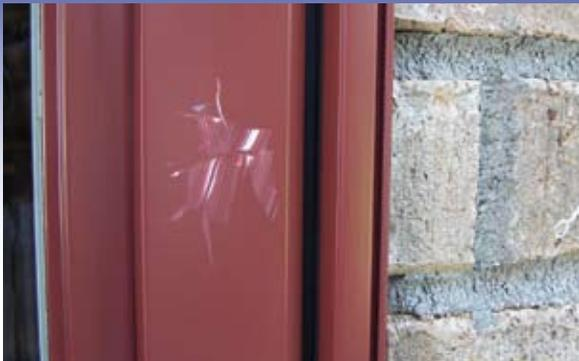
Large scrape on a casement window before being touched up. For repair on a larger area the foam brush technique usually provides the best results.
