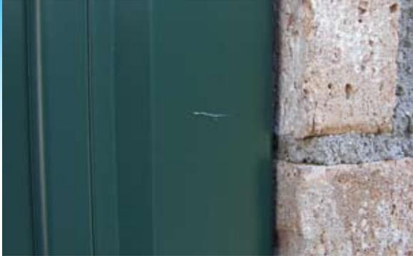
A small surface scratch shown on a picture window before being touched up using the applicator brush (included with the bottle of touch-up coating).
