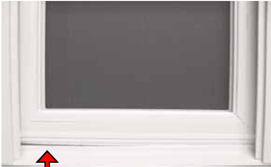
Inadequate Bulb Seal Compression
