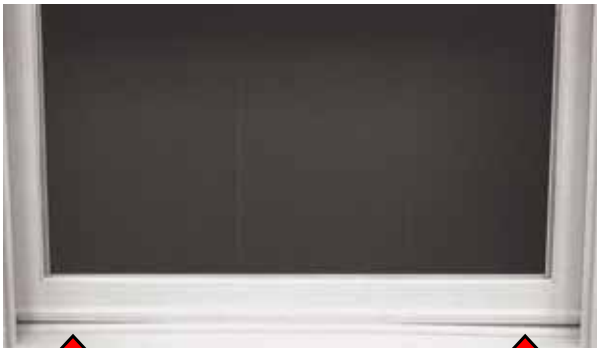
Inadequate Bulb Seal Compression
