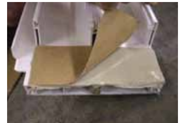
Correct placement of reinforcement.
